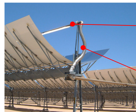
CSP - Solar Troughs
